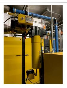
Air Main Charging Valve and Filter supports
