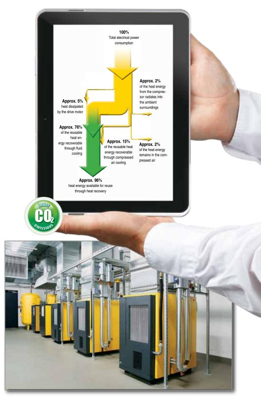
Air-cooled, fluid-injected screw compressors with internal heat exchangers and controls to tap into the thermal energy of the cooling fluid. The additional ducting removes the hot air that was not rejected by the hot water recovery system.
