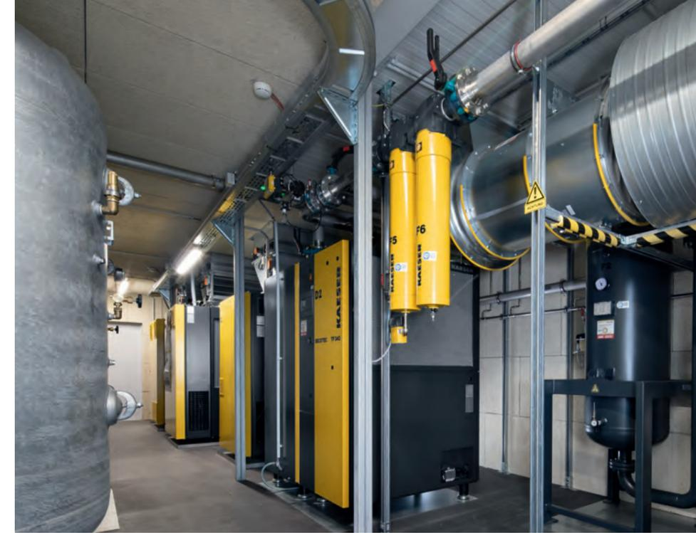
*The container housing the compressed air system has been completely lined with sound insulation mats to comply with sound emission limits.*
