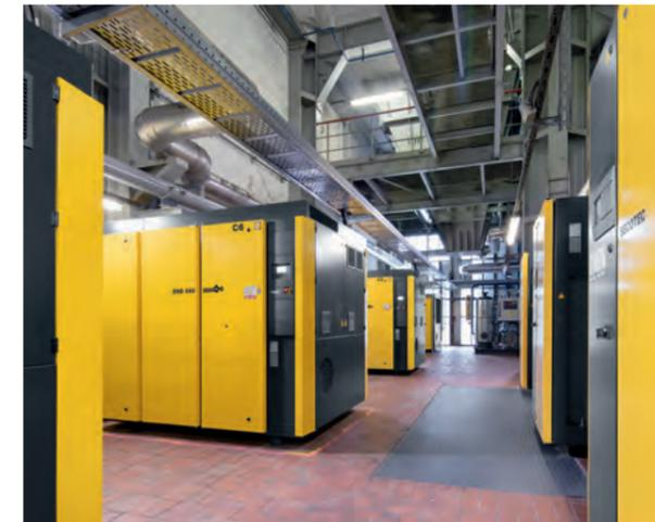
*A total of four rotary screw compressors with IE4 drive motors and the energy-saving SIGMA PROFILE operate in the compressed air system.*
