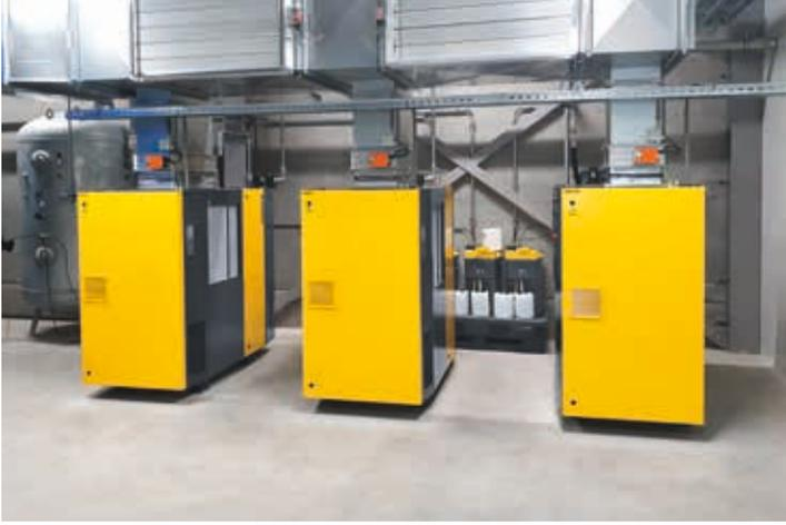
**KAESER ASD 40 T rotary screw compressors with heat recovery.**
