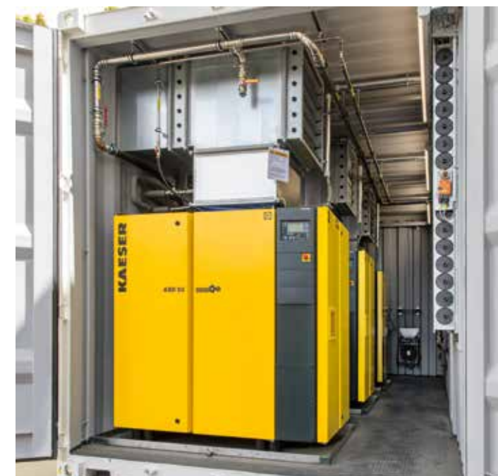
The three ASD 50 rotary screw compressors are installed in an enclosure along with a SIGMA AIR MANAGER 4.0 master controller, which controls the entire system at the highest levels of efficiency and in constant contact with the KAESER Service Center.
