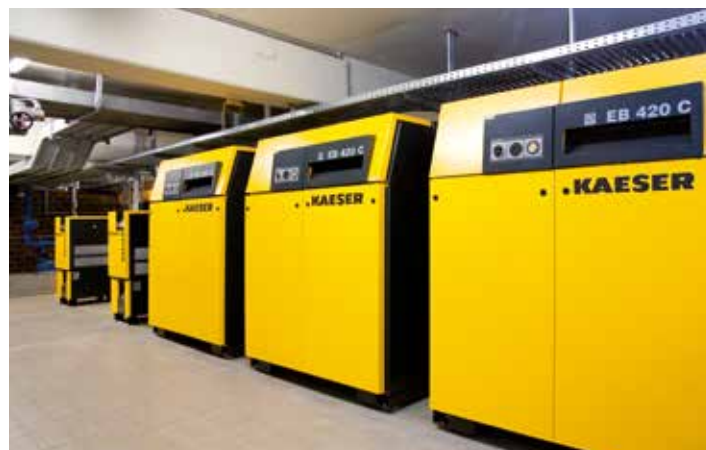
In the Jägersburg waterworks of the Wasserbeschaffungsverband Riedgruppe Ost, KAESER rotary blowers are coordinated and regulated by the central control system, ensuring the safe, efficient backwashing of the sand filters
