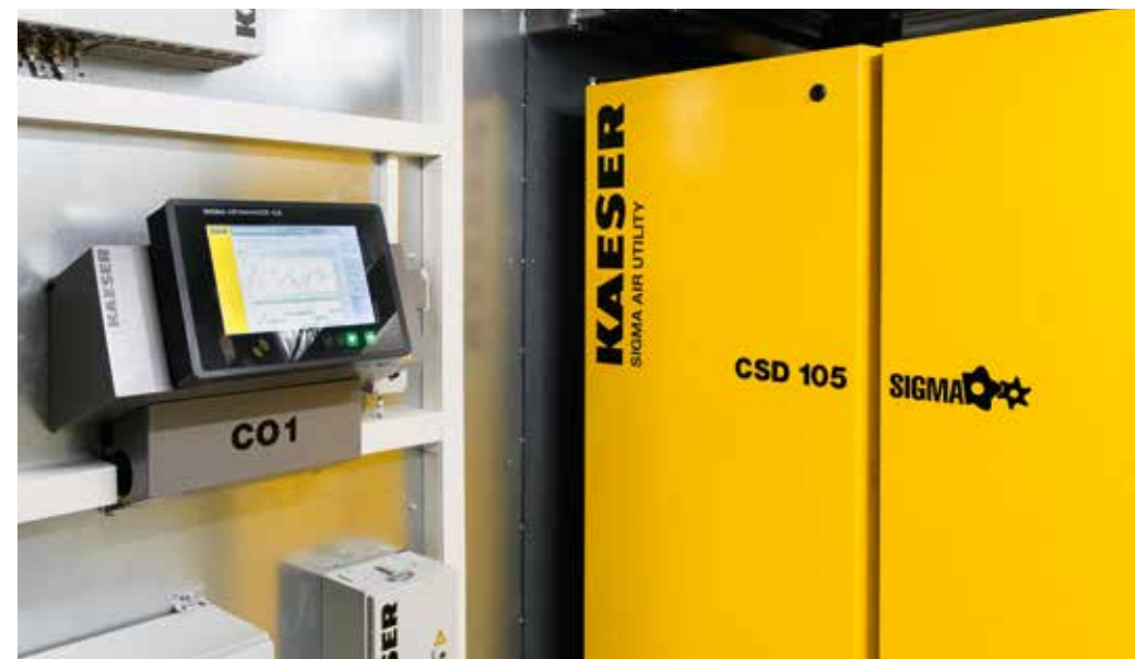
The SIGMA AIR MANAGER 4.0 manages the compressed air supply
