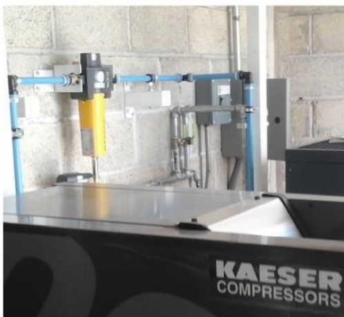
Rigid Pipe Supports with Flexible Connection at Discharge
