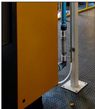
Rigid Pipe Supports with Flexible Connection at Discharge
