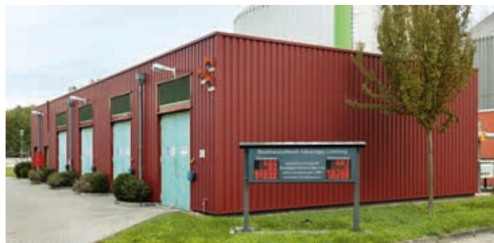
The illuminated panel shows the current values of the energy produced from the wastewater sludge.
