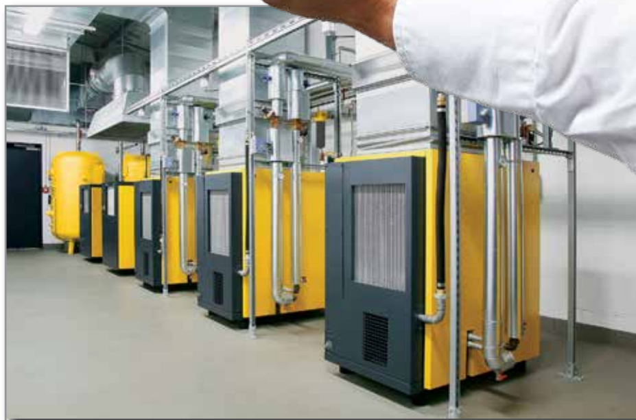
Air-cooled, fluid-injected screw compressors with internal heat exchangers and controls to tap into the thermal energy of the cooling fluid. The additional ducting removes the hot air that was not rejected by the hot water recovery system.
