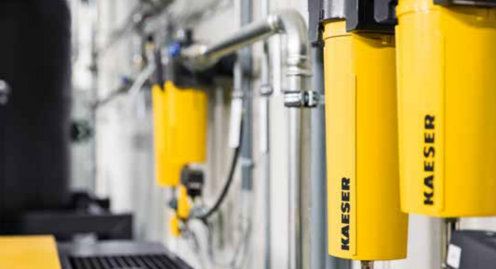
Refrigerated dryers of types TL 1301 and ABT 25, active carbon absorbers, microfne upstream filters, downstream filters for achieving Particulate Class 1 (as per ISO 8573-1) and several other filter devices ensuring the high quality of the compressed air.
