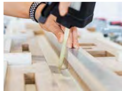
...or applying multi-component adhesive.
