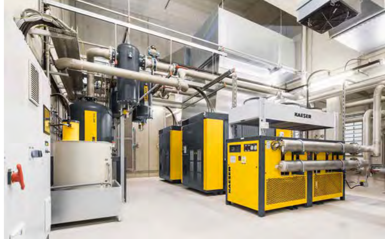
Refrigerated dryers of types TL 1301 and ABT 25, active carbon absorbers, microfne upstream filters, downstream filters for achieving Particulate Class 1 (as per ISO 8573-1) and several other filter devices ensuring the high quality of the compressed air.
