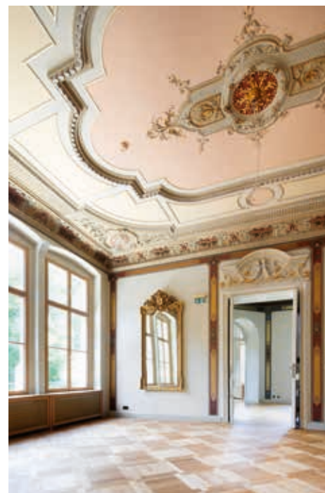
The stucco ceilings, as well as the wall and ceiling murals, had to be exposed and restored throughout the residence.
