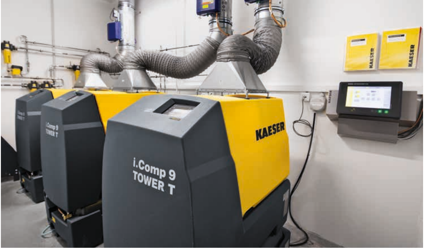
Three KAESER i.Comp 9 Tower packages ensure the large laboratory never goes without compressed air.
