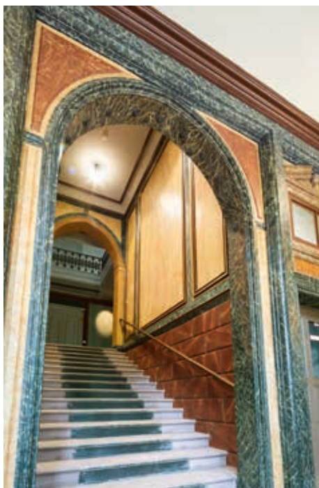
During the renovation, great care was taken to ensure that the historical fabric of the building was preserved.
