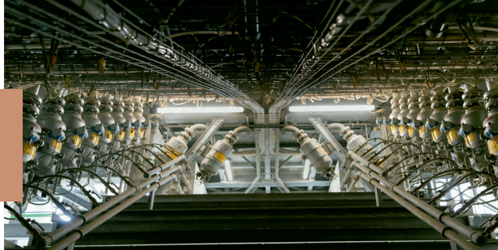
Compressed air distribution below the combustion chamber.
