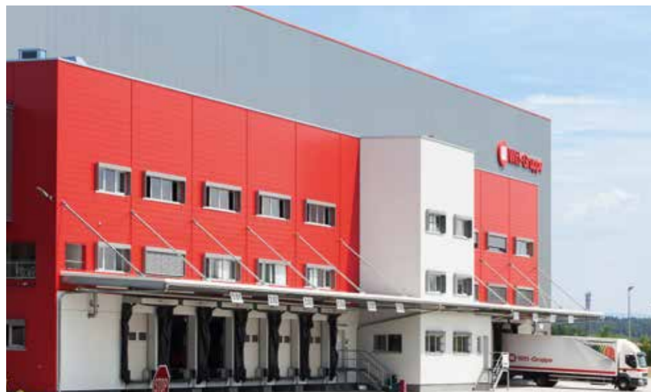
The logistics center in Weiden-Brandweiher
