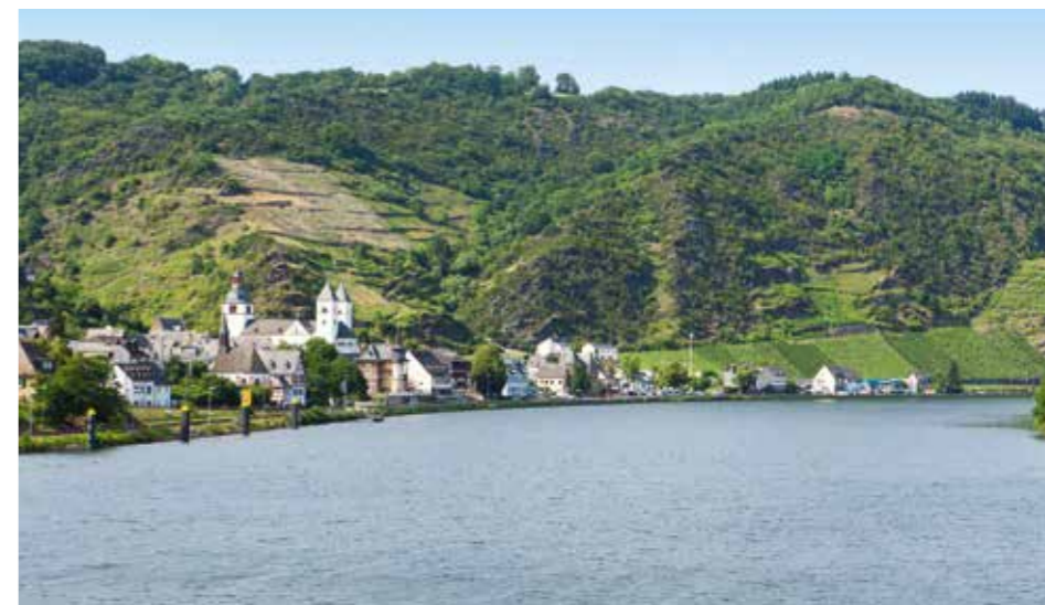
The Treis-Karden wastewater treatment facility (at left; above: Karden district with the St. Castor collegiate church) installed a new KAESER screw blower with excellent results
