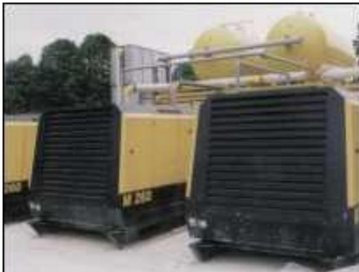
***Four Kaeser diesel-driven portable compressors of the type Mobilair 260 provide emergency backup. In the background can be seen the two containers (with air receivers) that house the Kaeser DSD 201 peak load compressor, the master controller and the air treatment components.***
