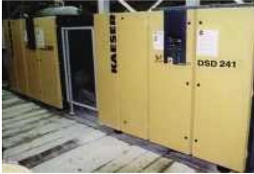
***Screw compressor packages installed underground to supply the base load***
