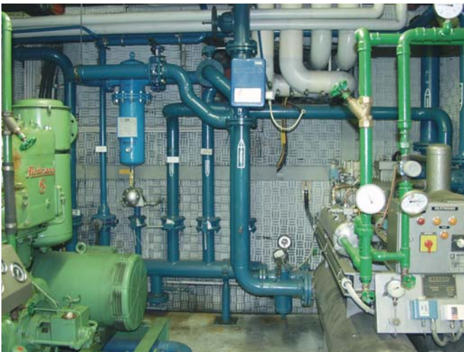
Fig. 6: Well-cared for but no longer up-to-date; the air system installed in an automotive production facility before modernisation
