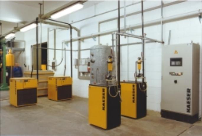
Two smaller KAESER SK screw compressors (to the left) generate the control air at 6 bar. The Vesis master controller (right) ensures even loading of the compressors, automatic control, monitoring and maximum availability of the compressor packages.
