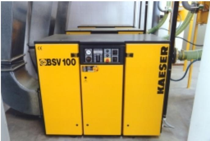
Three KAESER BSV screw vacuum pumps supply the factory with the vacuum required.
