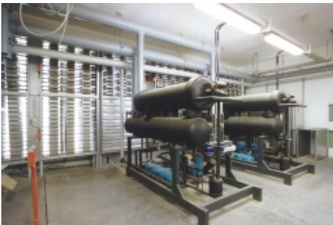
Two from altogether four refrigeration dryers of the station. The large-scale installations of the type Kaeser TL 7300 are responsible for the air treatment.
