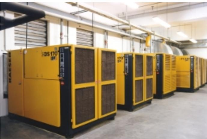
Seven larger KAESER FS, ES and DS screw compressors feed a 5 bar air main with the necessary compressed air.
